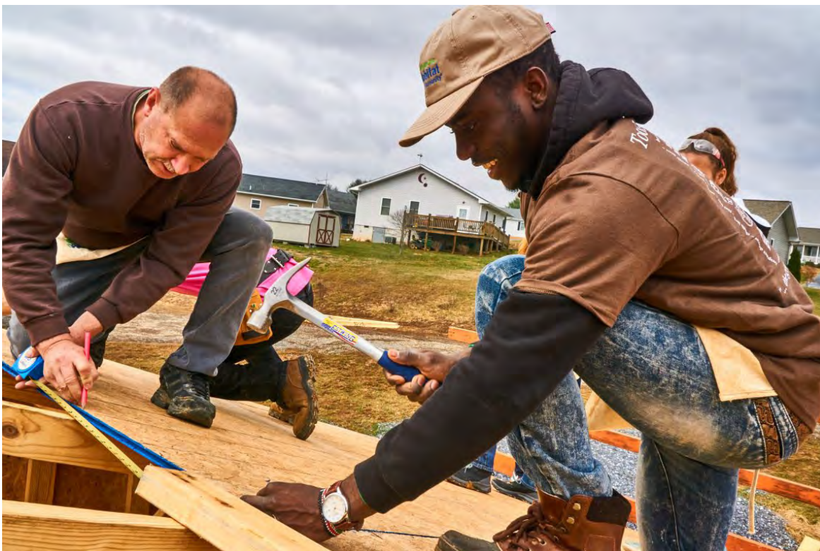
William Baya '22 works on a Habitat for Humanity project.
